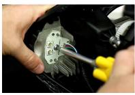
4. Using the alignment tabs, place the new board into place and replace the original T-20 screw. Next, replace the black alignment bracket using the original T-15 screws. DO NOT OVERTIGHTEN.
